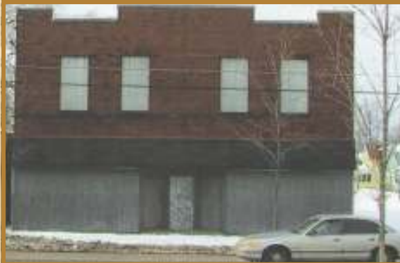
525 Eastern Ave prior façade renovations
