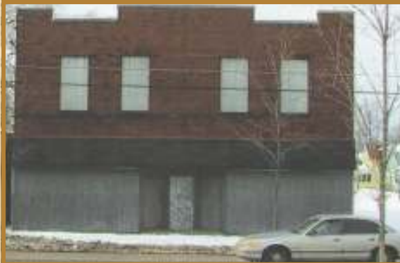
525 Eastern Ave prior façade renovations
